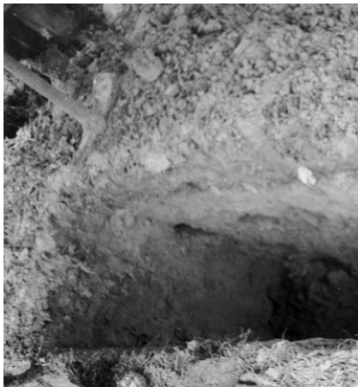
Colombia. 2001. Excavating initial trenches. photo by EAAF
